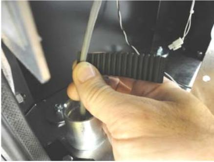
**B** - Continue to wrap cable until diameter is about the size of the inside of the conduit (3/4").
