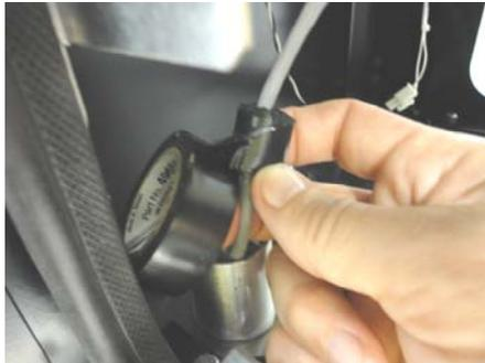
**D** - Push cable and seal down into conduit fitting so that top of gasket is 1-1/4" deep into the conduit.
