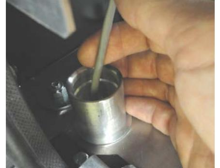
**E** - View of Ethernet cable and conduit before potting. (Picture shows fitting outside of dispenser.)
